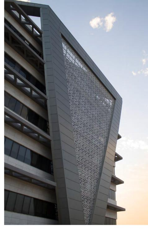
Ramallah is known for its mediterranean climate with cold winters and long, warm and dry summers with average daily temperature above 25°C, which is why the Qbiss One facade system was also the best choice thanks to its insulation properties. With mineral wool insulation it can achieve a high thermal insulation level with U values up to 0.16 W/m<sup>2</sup>K and contributes to thermally pleasant and stable interior climate.
