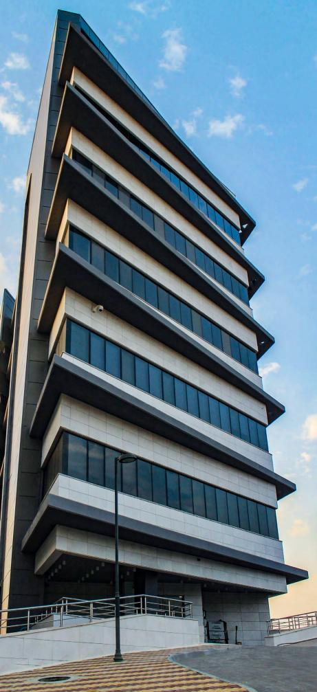
The dynamic of the horizontally assembled façade is created by alternating local stone cladding and slightly overhanging assembled Qbiss One elements.
